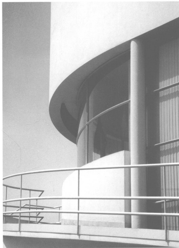
1 An identity based on the spatial and formal qualities of masonry structure. Borges & Irmão Branch Bank, elevation detail
